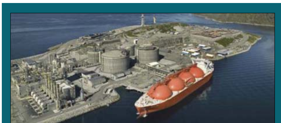
Hammerfest LNG is shutting down until November for extensive upgrading and maintenance. Photo by Eiliv Leren, StatoilHydro.
